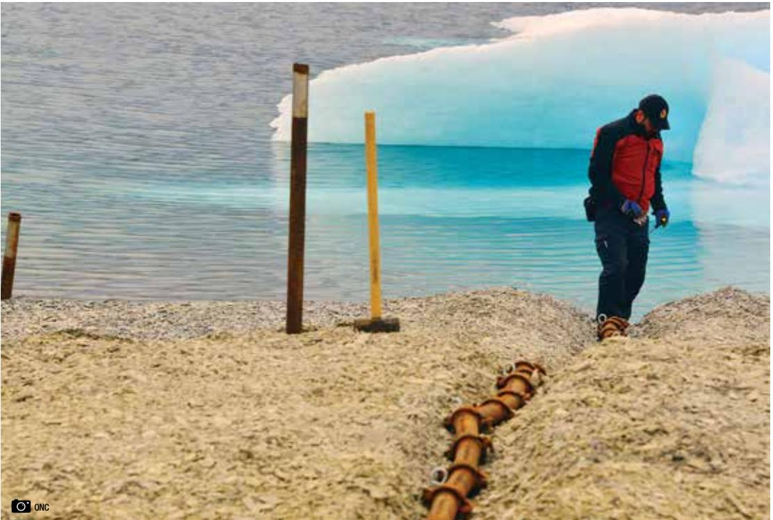
Figure 3: Subsea cable protection from sea-ice on Devon Island.
